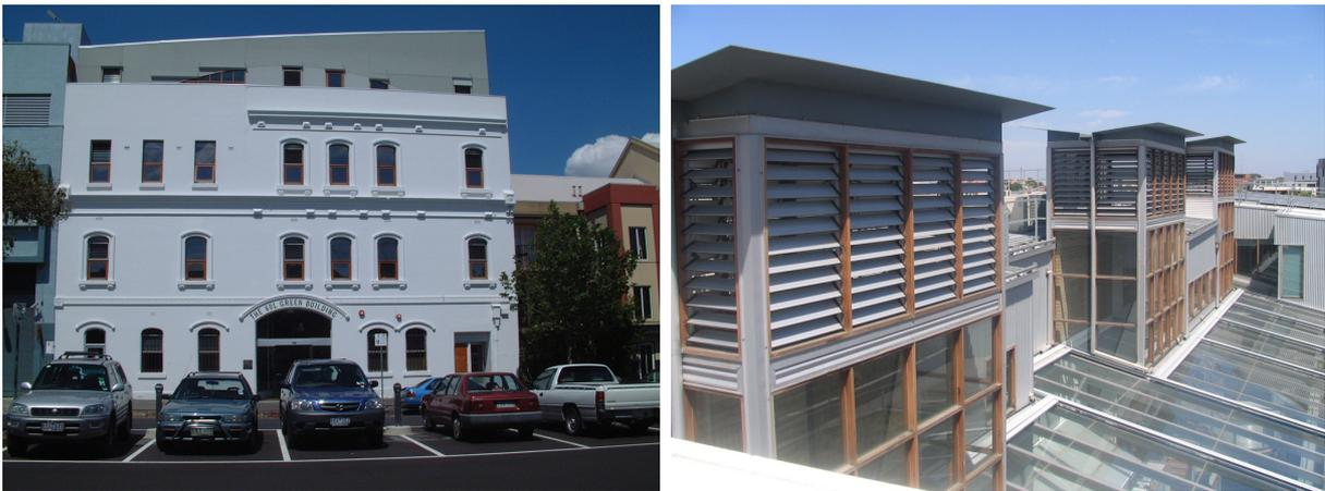
Fig C.8 Front façade and thermal chimneys of 60L Green Building (Source: ACF)
